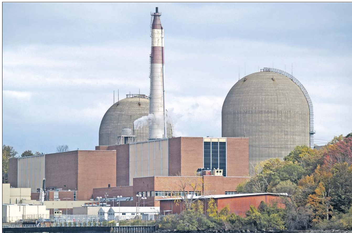
A pending deal for the aging Indian Point nuclear power plant could end up costing customers via a hike on their electric bills. Photo by Bloomberg News
